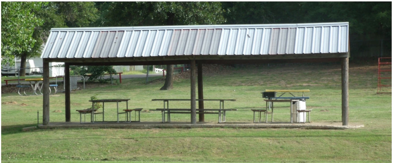
The pavilion at Optimist Park
